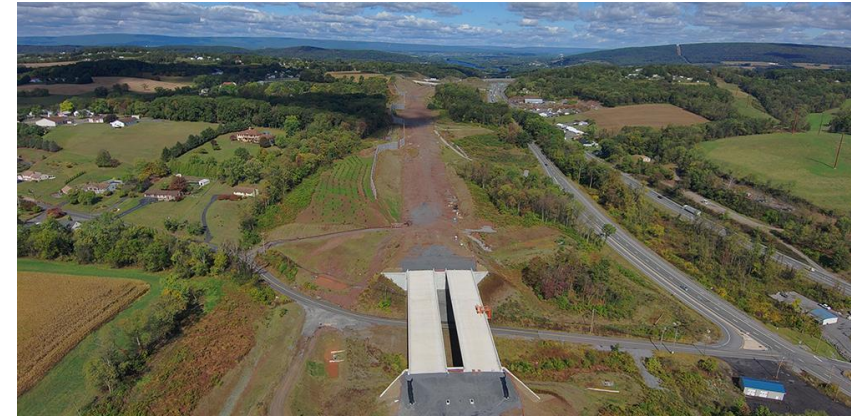
Looking north towards Winfield interchange
