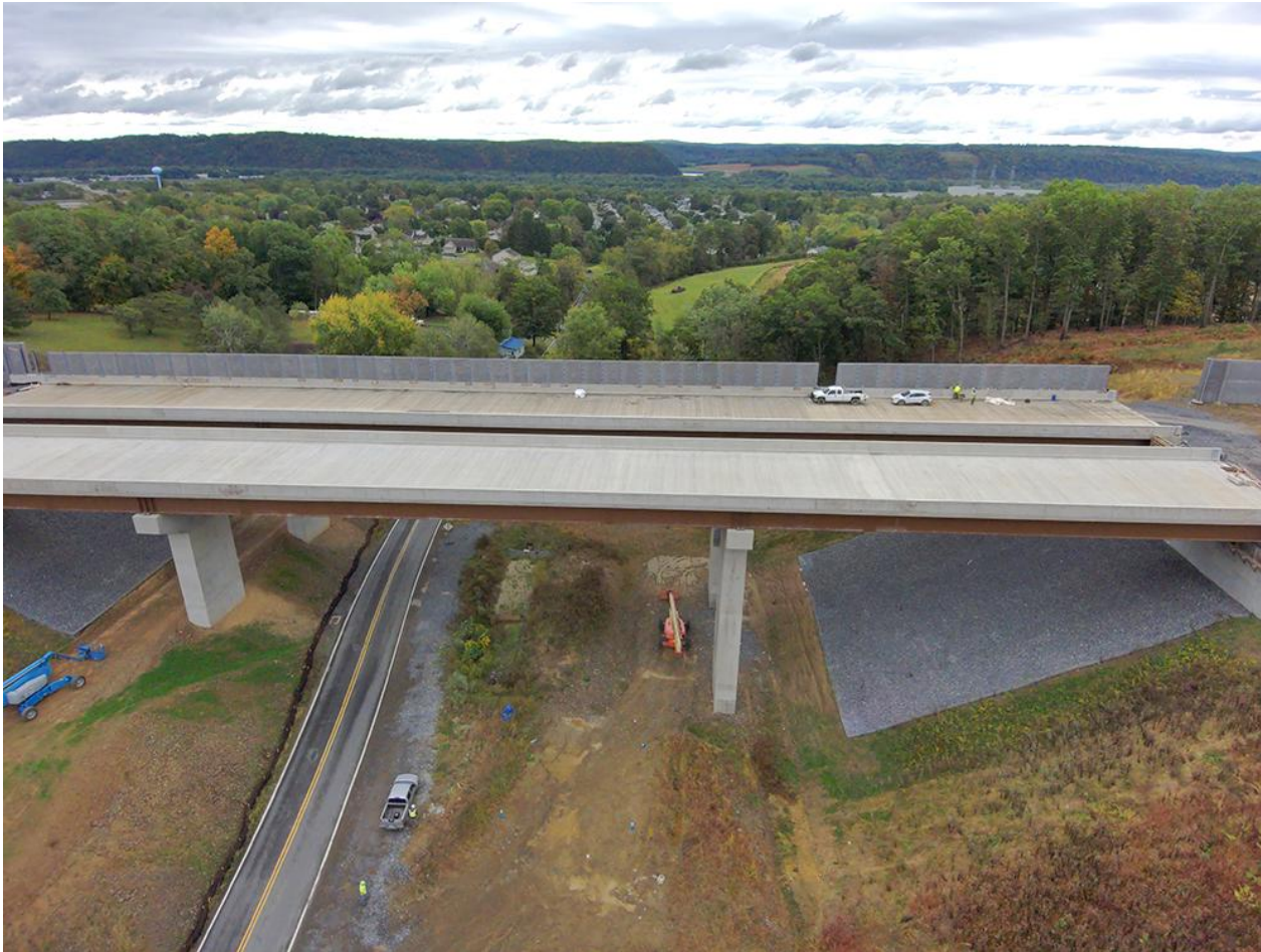
Looking southeast at CSVT bridge over 11 th Ave.
