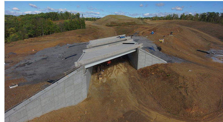
Looking north at CSVT bridge over PA 61 Connector
