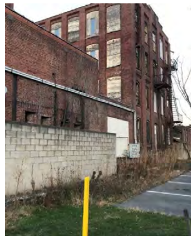
Future site of hotel on W Walnut Street
