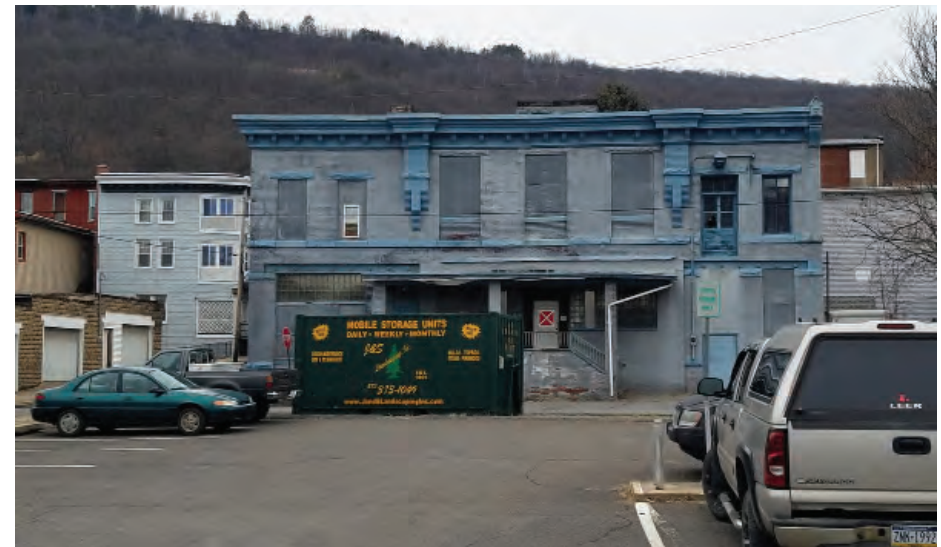
2020 view of F&S Brewery building
