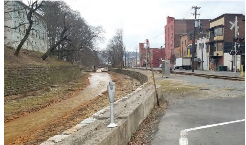
Shamokin Creek adjacent to downtown building
