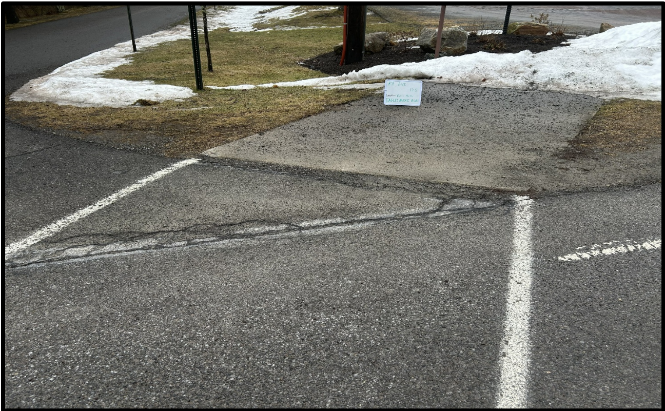
BELOW: Pennsylvania Avenue #125
