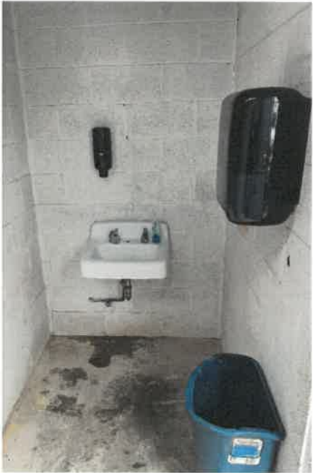
Photo 3 (above): Sink in the interior of the women's restroom.
