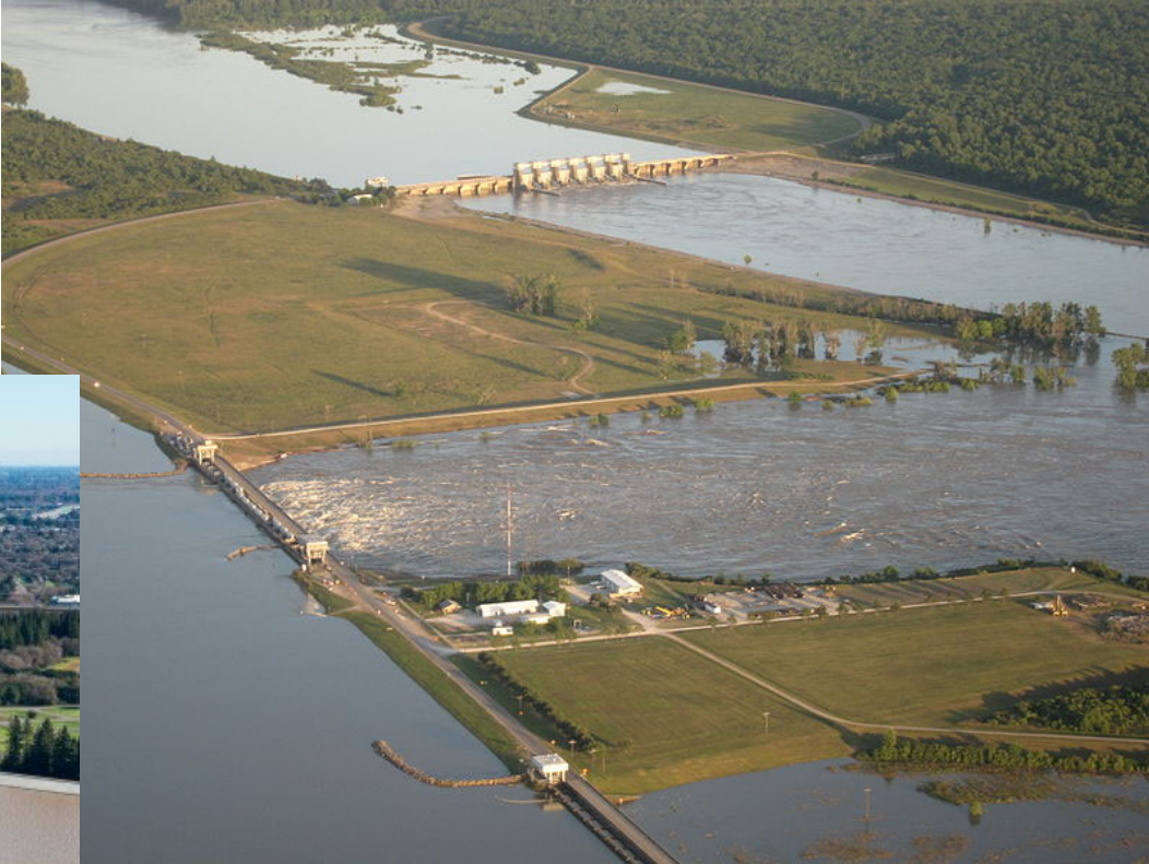
USACE – Mississippi Old River Control Structure Louisiana
