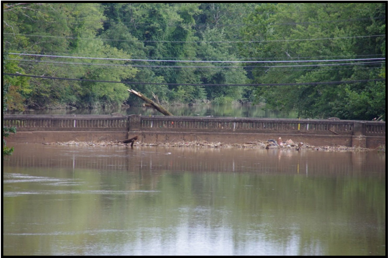
Figure 4.2 – Red Mill Road Bridge (2011 Event Facing Upstream)
