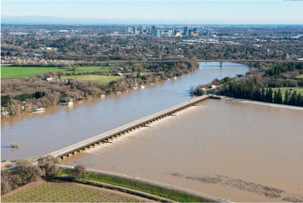
US Bureau of Reclamation – Yolo Bypass Habitat Restoration/Fish Passage Project Sacramento, CA
