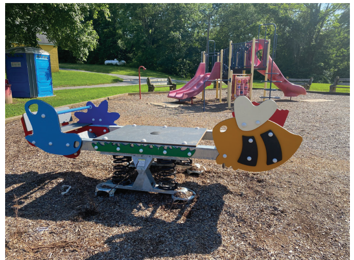
Marysville Borough Park Rehabilitation - Phase II Community Development Block Grant (CDBG) New ADA playground equipment installed.
