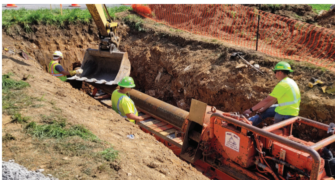
SR 44 watermain replacement in Limestone Twp.
