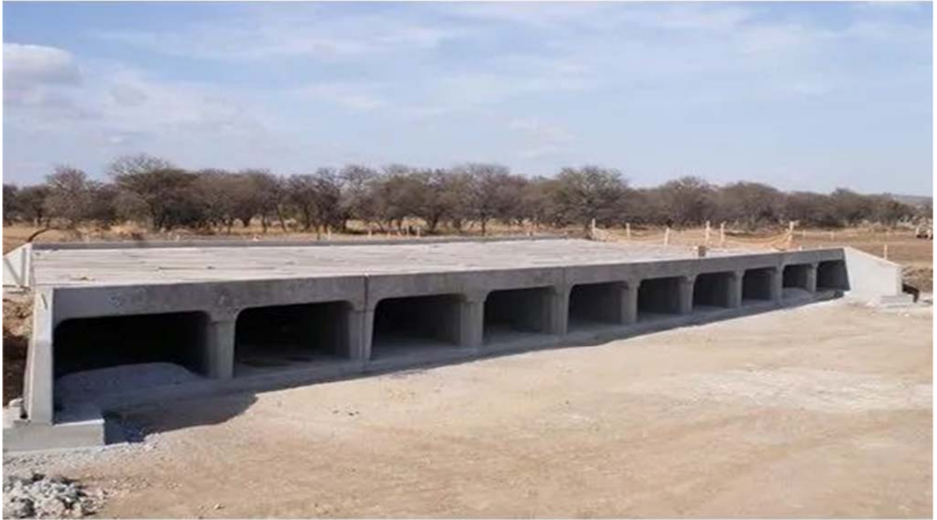
Figure 2.5 – Typical Concrete Box Culverts in Series
