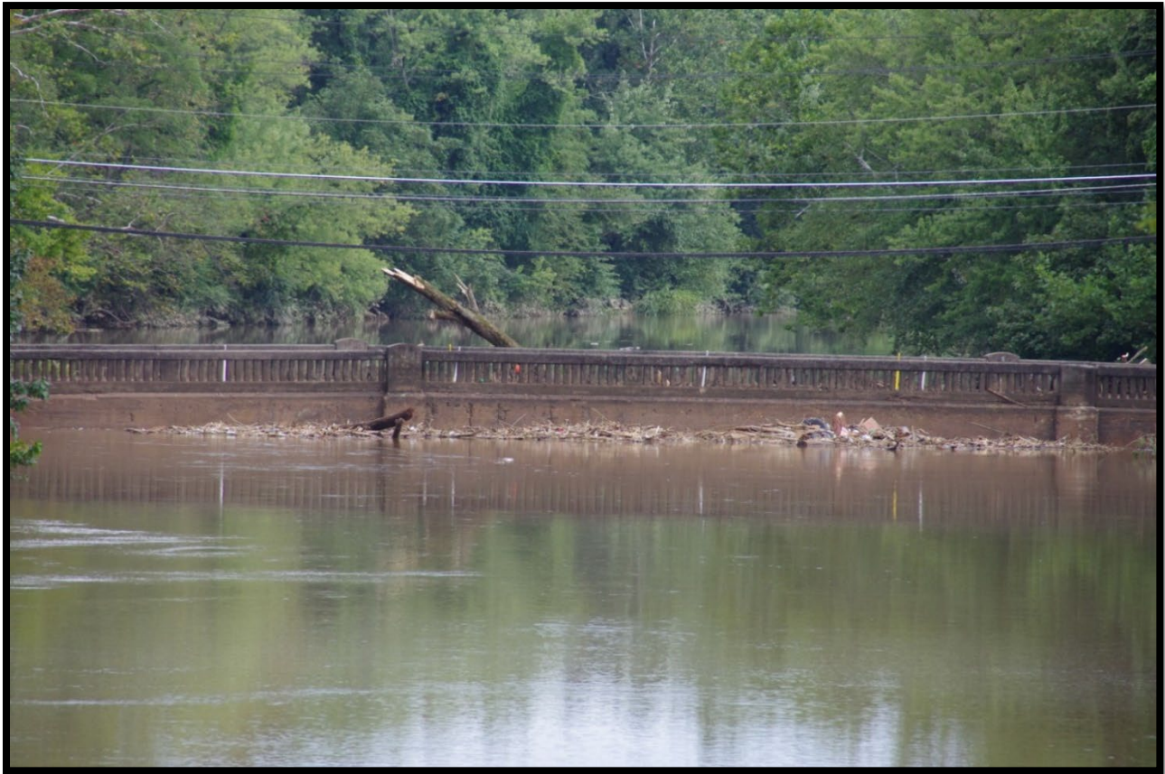
Figure 4.2 – Red Mill Road Bridge (2011 Event Facing Upstream)
